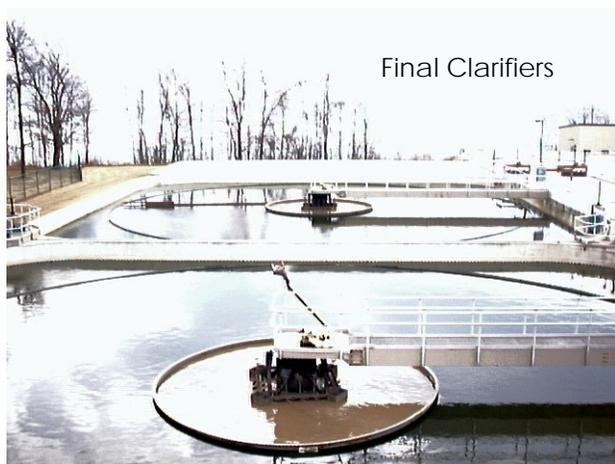
organisms in the system. A portion of activated sludge, known as waste activated sludge, is pumped to a point upstream of the primary clarifiers where it is co-mingled with the raw wastewater and removed in the primary clarifier. Waste activated sludge is removed from the system to maintain the proper population of micro-organisms to provide the most effective treatment.
